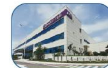
Qingdao Sino-German factory (Electric water heater)
